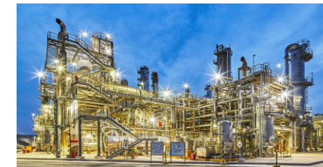
화공 (Chemical Plant)
