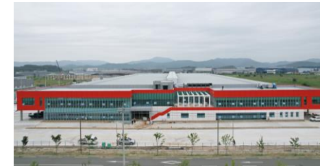
산업설비 (Industrial Facility)
