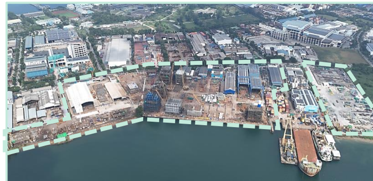
Gul Yard (Singapore) incl. 'Gul Yard 2' & '49 Gul Road' • 총 면적: 198,300 m 2 , 안벽길이: 680 m
